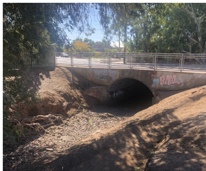
Bridge Upgrade - Before
