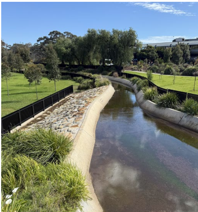
Glenside concrete swale
