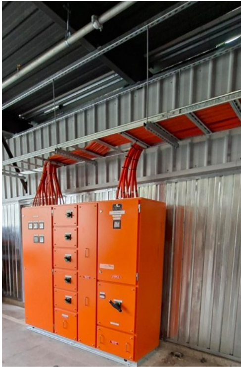
Evaporative plant works – Existing Market carpark level 2
