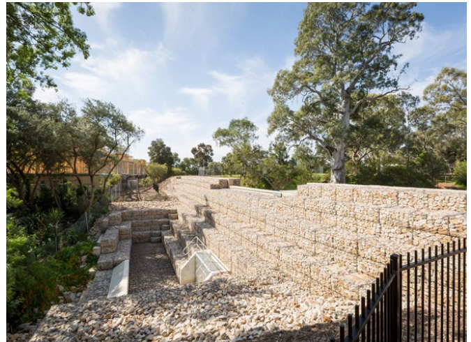
Ridge Park - Flood Control Dam
