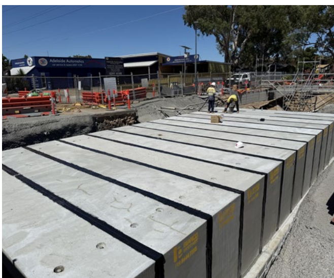
Lower Brown Hill Creek Upgrades - culvert installation
