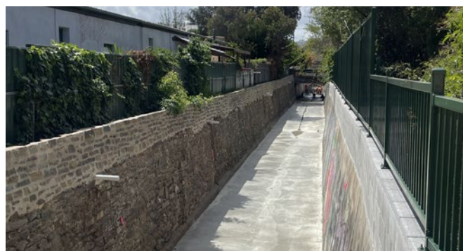
Leah St to Ethel St - Raised channel walls
