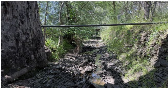
Orphanage Park - Existing Channel
