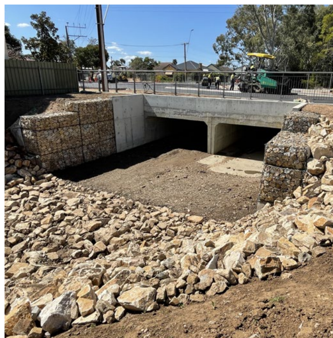
Bridge Upgrade - After
